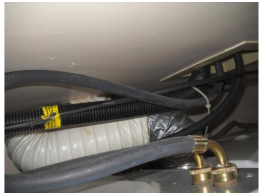
6. Dryer vent is plastic flex.
