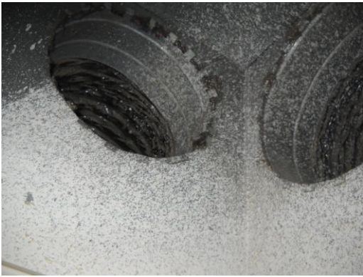
11. This supply had a pressure pan reading of over 6 pascals. All supplies need sealing at the ceiling.
