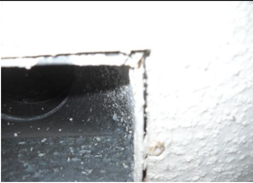
11. This supply had a pressure pan reading of over 6 pascals. All supplies need sealing at the ceiling.
