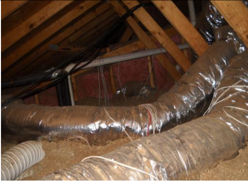
7. Insulation in attic is blown cellulose, average 7 inches.
