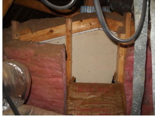
10. Air infiltration from attic at recessed lighting.
