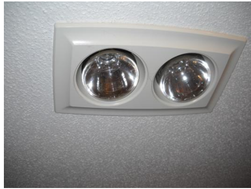
10. Air infiltration from attic at recessed lighting.
